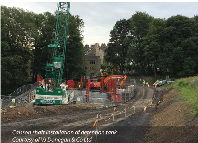
*Caisson shaft installation of detention tank
