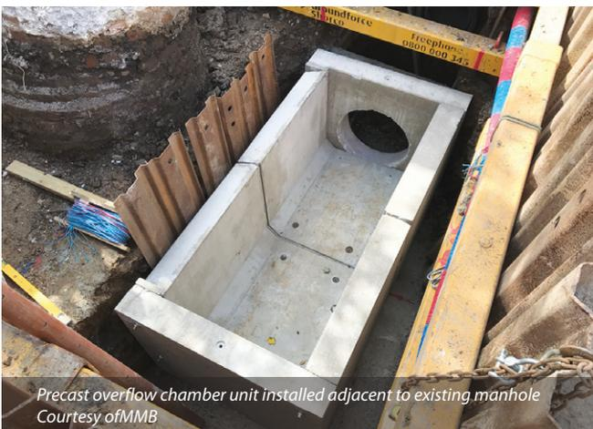
*Precast overflow chamber unit installed adjacent to existing manhole
