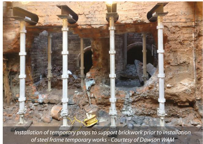
Installation of temporary props to support brickwork prior to installation of steel frame temporary works - Courtesy of Dawson WAM
