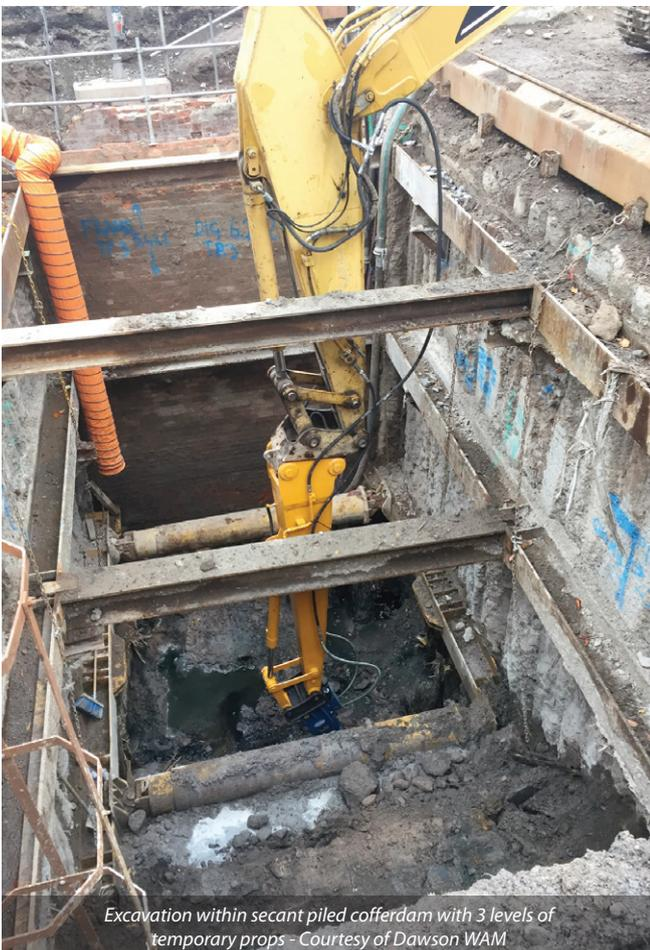
Excavation within secant piled cofferdam with 3 levels of temporary props - Courtesy of Dawson WAM
