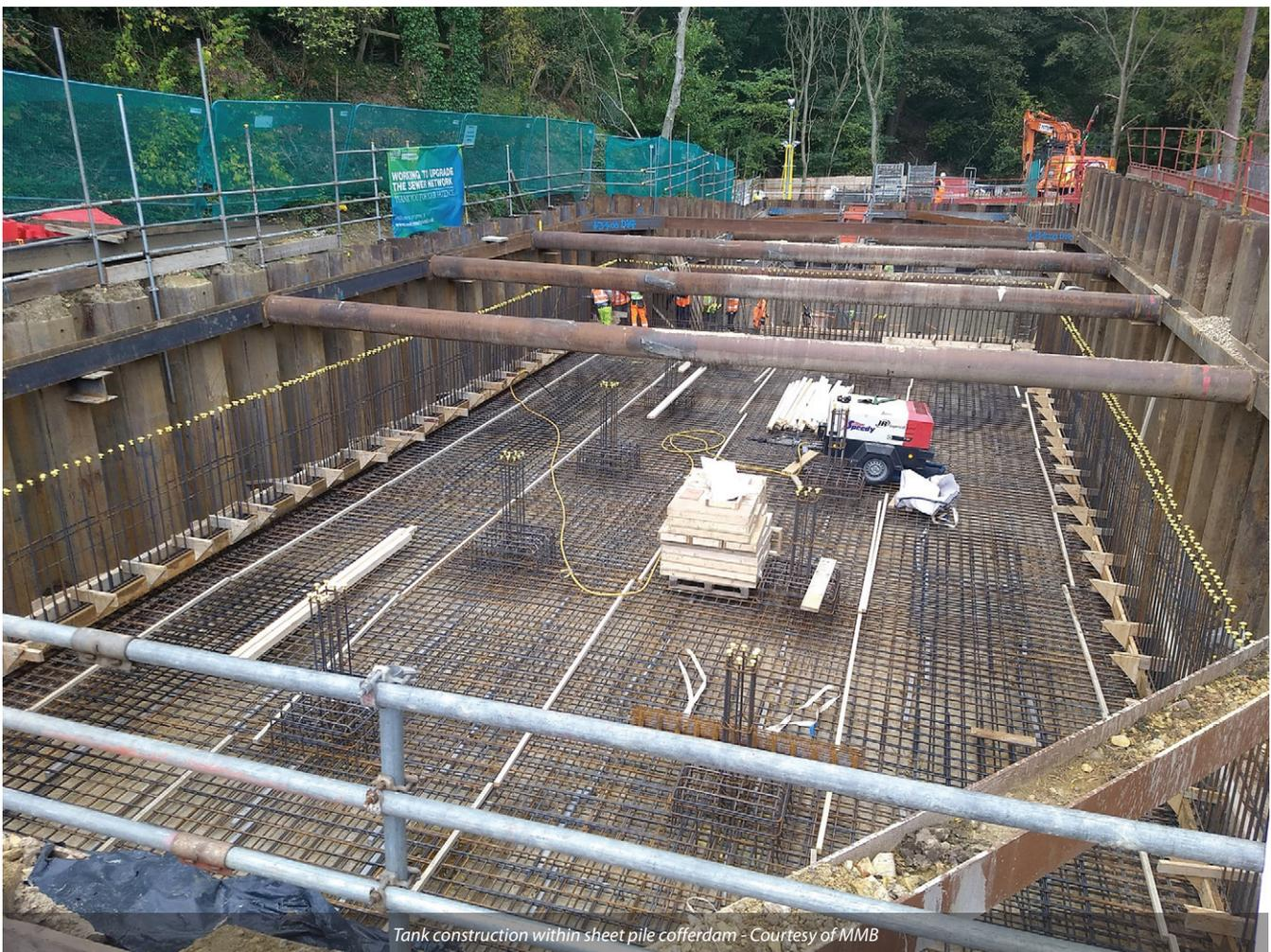
Tank construction within sheet pile cofferdam - Courtesy of MMB
