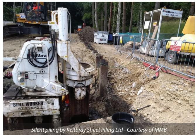
*Silent piling by Keltbra Sheet Piling Ltd - Courtesy of MMB*
