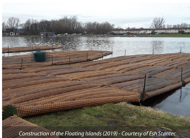
Construction of the Floating Islands by Biomatrix (2019) Courtesy of Esh Stantec
