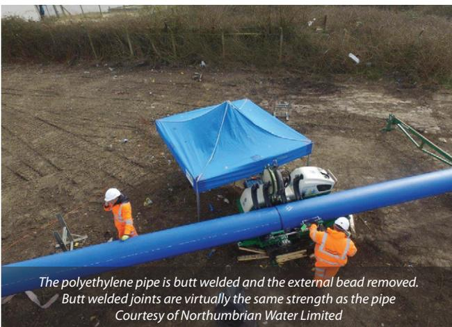
The polyethylene pipe is butt welded and the external bead removed.
