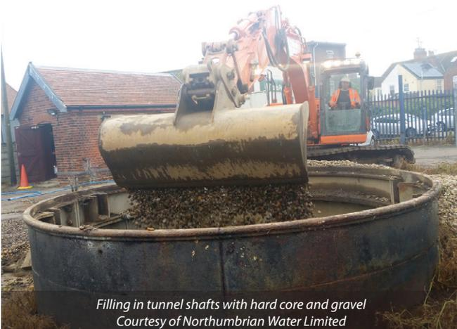
Filling in tunnel shafts with hard core and gravel
