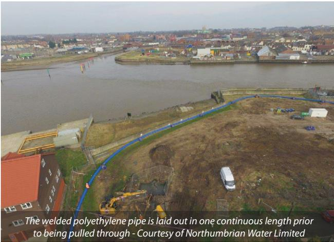
The welded polyethylene pipe is laid out in one continuous length prior to being pulled through - Courtesy of Northumbrian Water Limited
