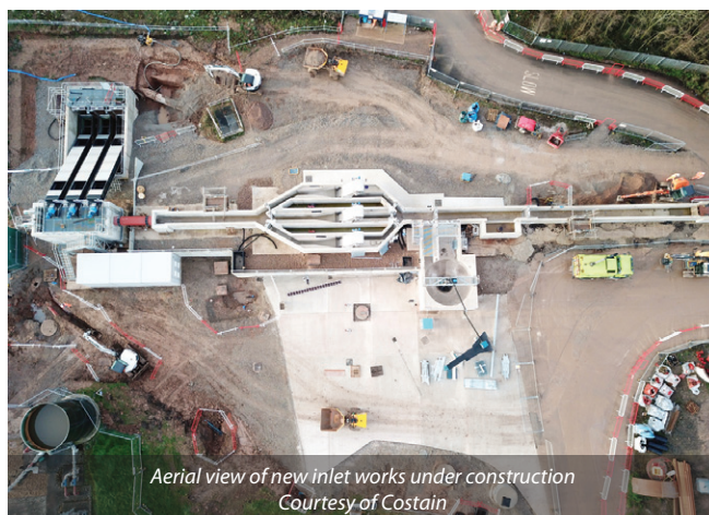
Aerial view of new screw pump station and inlet works under construction Courtesy of Costain
