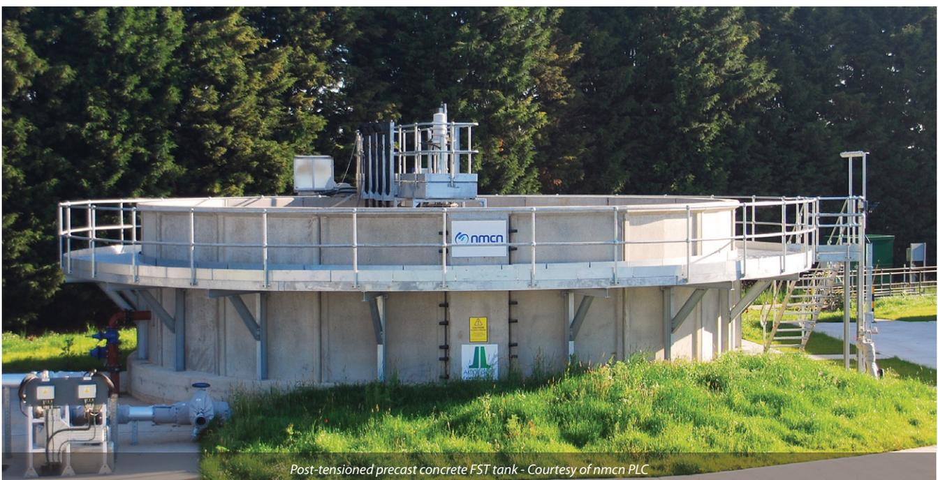
Post-tensioned precast concrete FST tank - Courtesy of nmcn PLC
