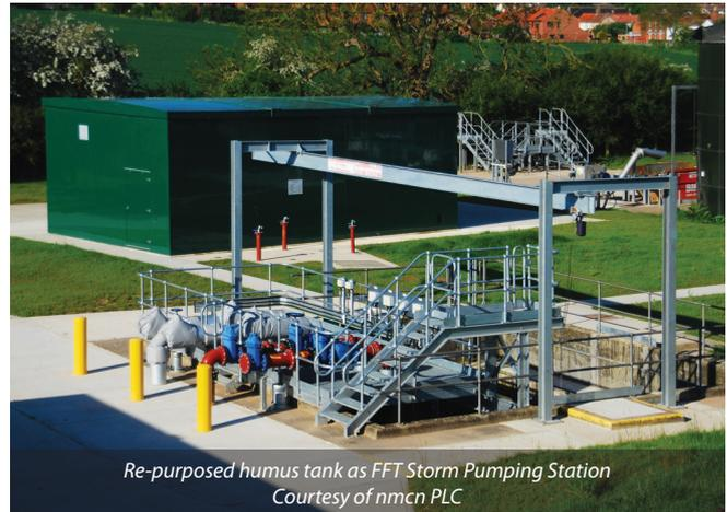
Re-purposed humus tank as FFT Storm Pumping Station
