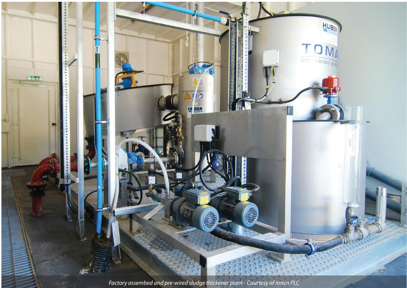
Factory assembled and pre-wired sludge thickener plant - Courtesy of nmcn PLC
