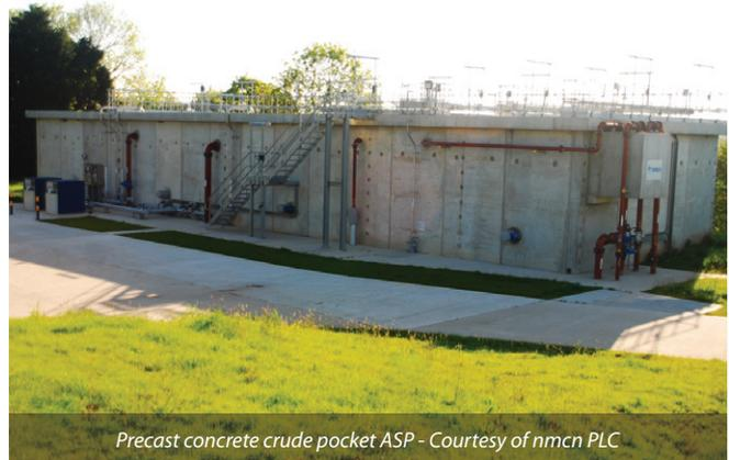
Precast concrete crude pocket ASP - Courtesy of nmcn PLC
