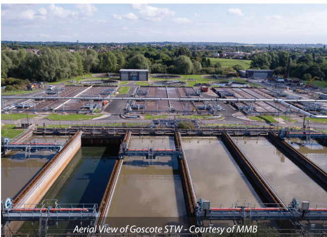
Installation of the IFAS Cages - Courtesy of MMB
