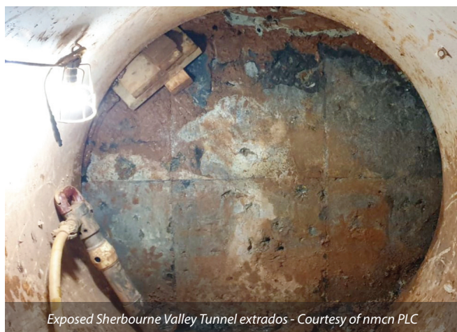
Coring through RC portal into tunnel - Courtesy of nmcn PLC
