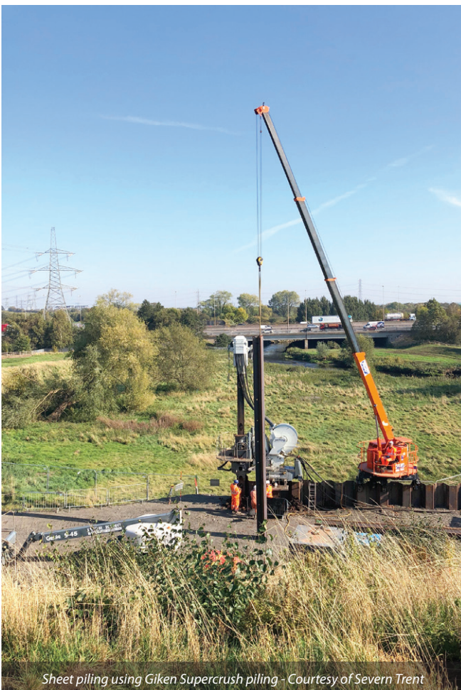
Haul road stabilisation - Courtesy of Severn Trent
