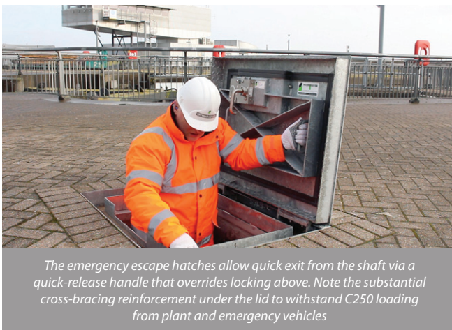
Technocover's access covers provide vital emergency escape through strategic shafts to the barrage gallery contained within the dockside to the substantial 16m-deep locks
