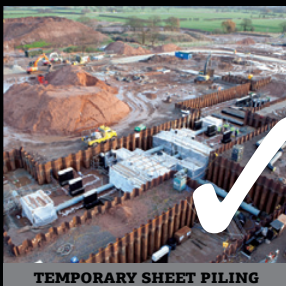
TEMPORARY SHEET PILING
