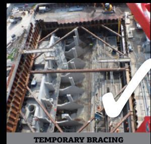
TEMPORARY BRACING
