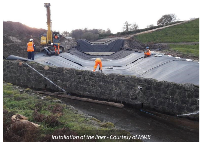
Weir cut off into the clay core - Courtesy of MMB
