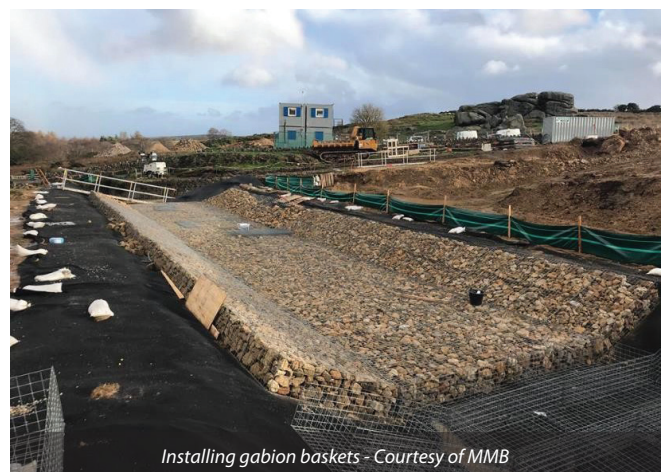
Installation of the liner - Courtesy of MMB
