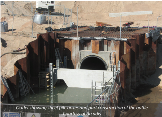
Pipeline pumping to the sea - Courtesy of Arcadis
