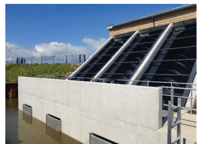
3 screw pumps supplied, installed and commissioned for a water drainage project
