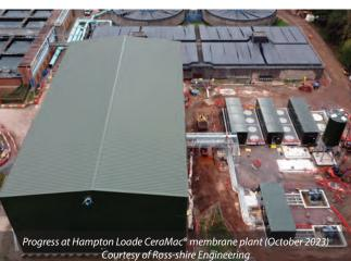
The CeraMac® solution was chosen as it provides an advantage over RGFs due to the robust physical barrier it presents against particulates. Due to the 0.1-micron pore size within the membrane, the CeraMac® process provides an absolute barrier against cryptosporidium oocysts and the clostridium perfringens bacteria that is present within the raw water at Hampton Loade WTW.
