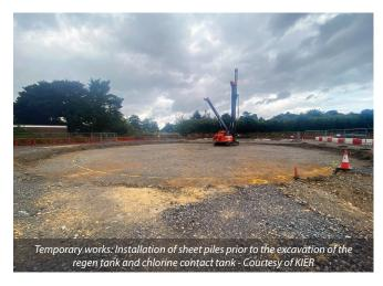
**Construction: ONGOING:** Construction activities have been progressing on site over the last year. The enabling works have included ground clearance and demolition of old buildings over the construction area. Foundation/piling work is also now complete in preparation for the above-ground structures which will progress on site at the back end of 2023.
