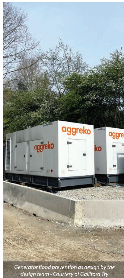
Aggreko duty, primary assist and secondary assist generators - Courtesy of Galliford Try
