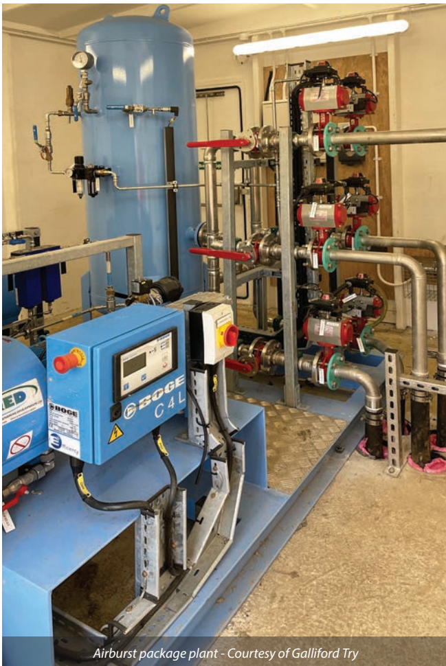
Airburst package plant - Courtesy of Galliford Try
