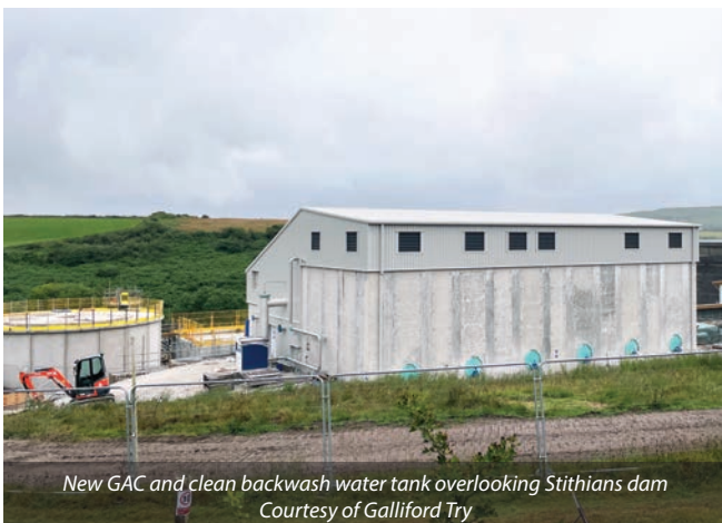
Clean backwash tank pump station - Courtesy of Galliford Try
