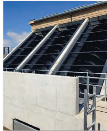
NEW MONKS FARM DRAINAGE PS 3 (No.) screw pumps supplied, installed and commissioned
