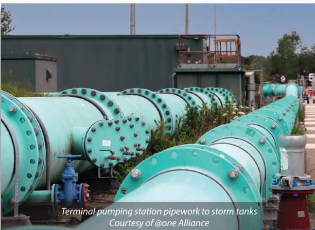
Construction of the two new storm tanks - Courtesy of @one Alliance
