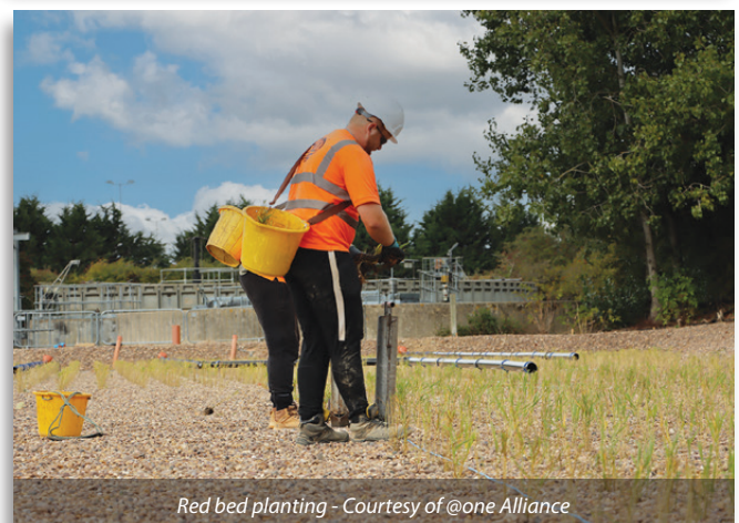
Preparing the ground for the reed bed - Courtesy of @one Alliance
