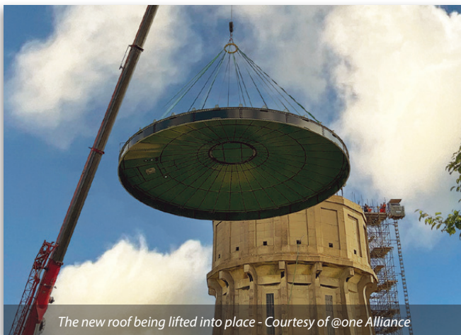
New roof ready to be lifted - Courtesy of @one Alliance
