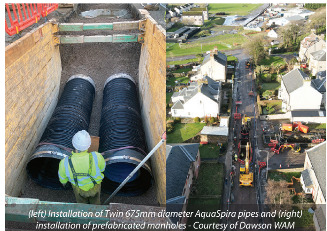
Storm separation pipework installation at Witchburn Courtesy of Dawson WAM
