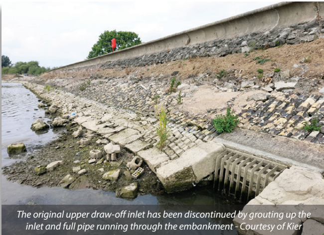
Decommissioning the original primary spillway with double concrete walled structure with brickwork fascias to match original spillway - Courtesy of Kier
