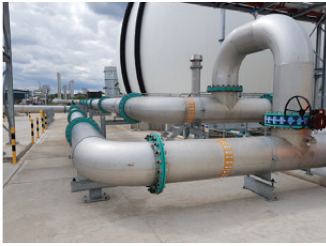
Biogas Pipework
