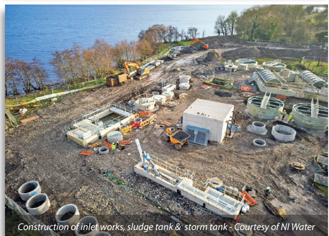
Aerial view of construction November 2023 - Courtesy of NI Water
