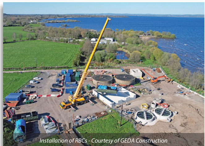
RBC reinforced concrete base - Courtesy of GEDA Construction
