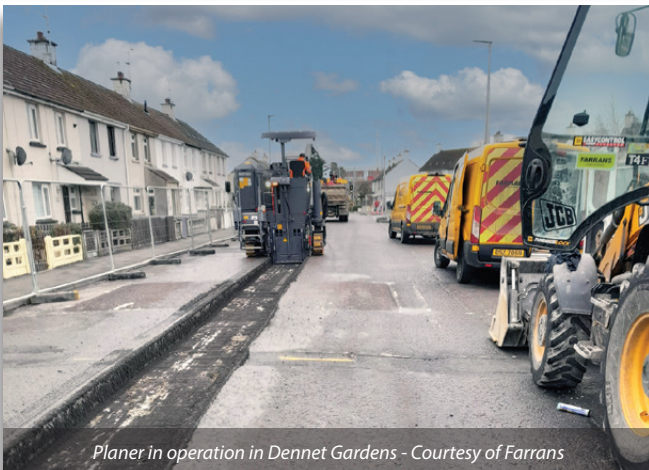
Planer in operation in Dennet Gardens - Courtesy of Farrans
