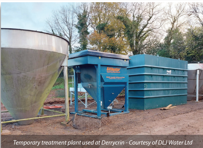
Derrycrin during construction (August 2023) - Courtesy of NI Water
