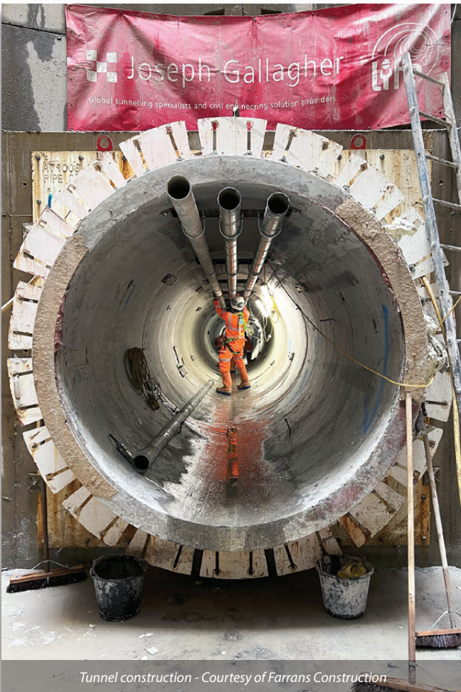
Pipe laying - Courtesy of Farrans Construction
