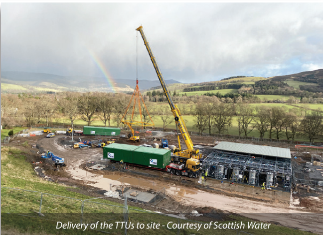
Delivery of the TTUs to site - Courtesy of Scottish Water
