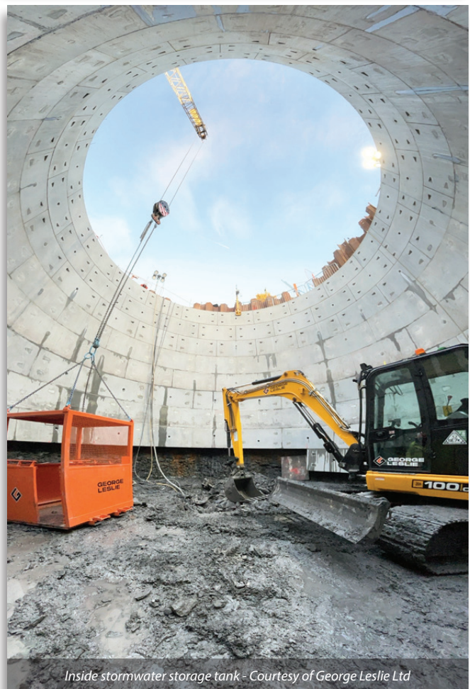
Site establishment - Courtesy of Whitehouse Studios
