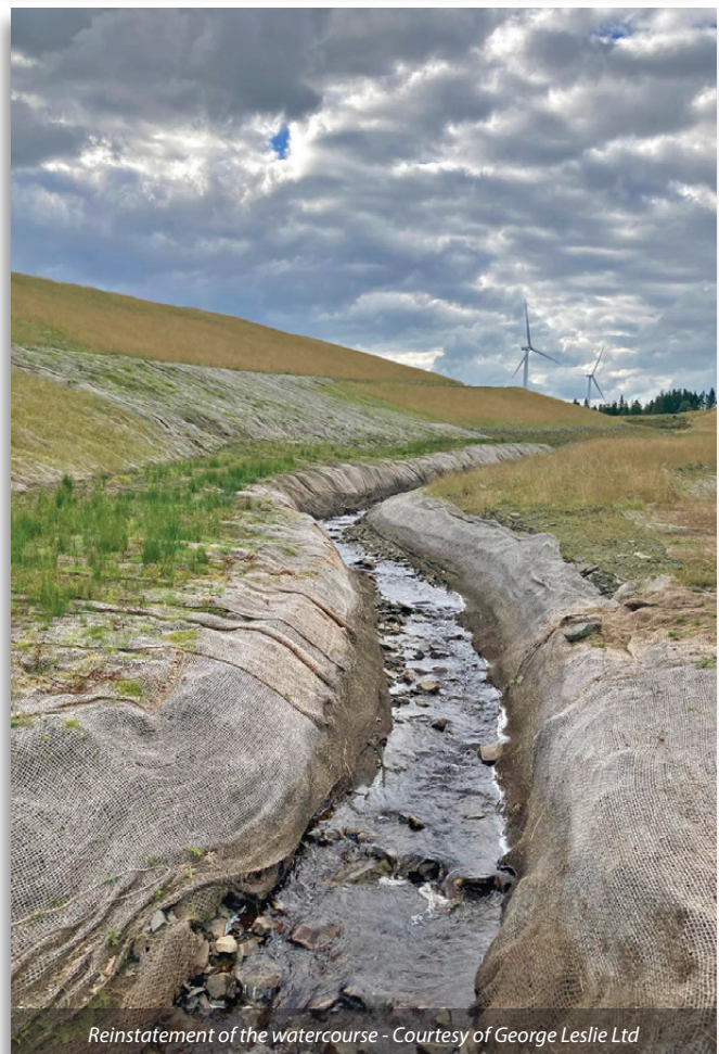
Reinstatement of the watercourse - Courtesy of George Leslie Ltd
