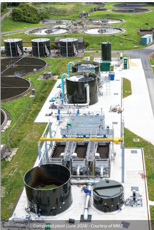
Construction progress (August 2023) - Courtesy of MMB
