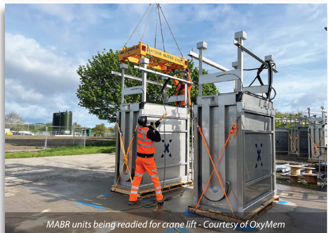
MABR steelwork - Courtesy of OxyMem
