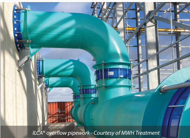
Witches Oak WTW site overview (May 2024) - Courtesy of MWH Treatment
