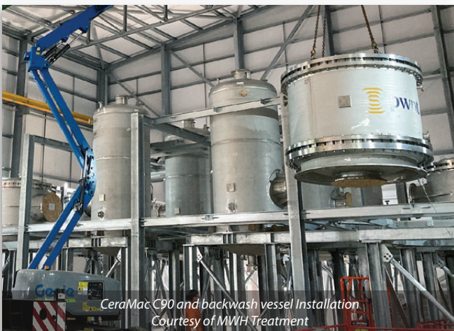
Membrane building Konecrane installation - Courtesy of MWH Treatment
