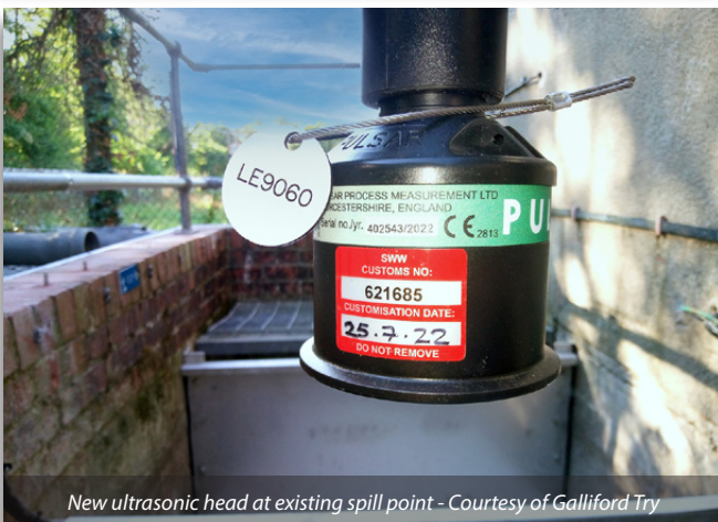
New ultrasonic head in existing tank - Courtesy of Galliford Try
