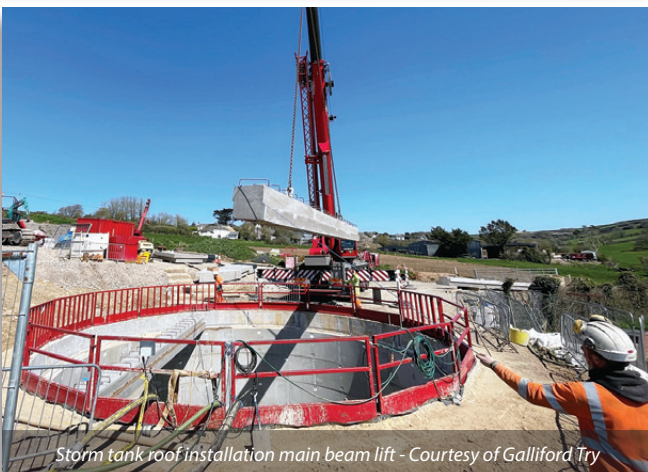
Installation of the precast concrete roof - Courtesy of Galliford Try
