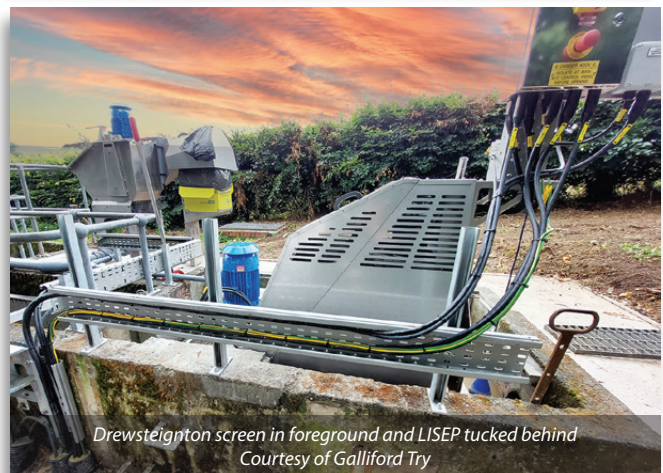
Moreleigh STW: New screen, LISEP and grit trap - Courtesy of Galliford Try
