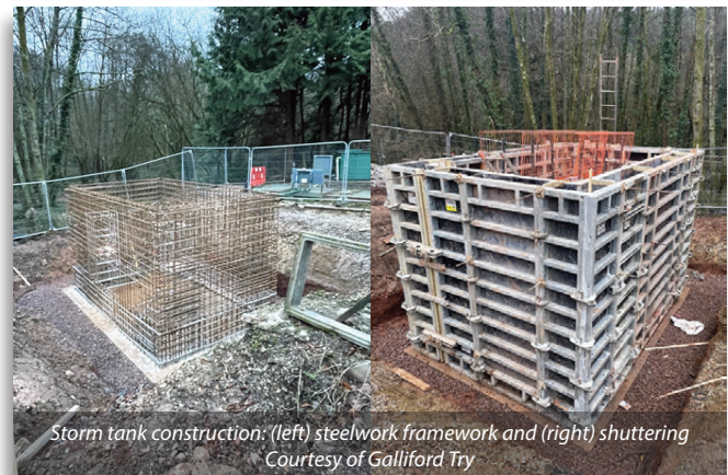
Shuttering and steelwork for tank base - Courtesy of Galliford Try
