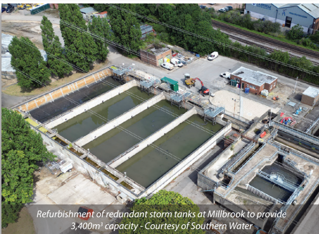
UV irradiation system at Millbrook (June 2024) post commissioning/FST under construction - Courtesy of Southern Water
