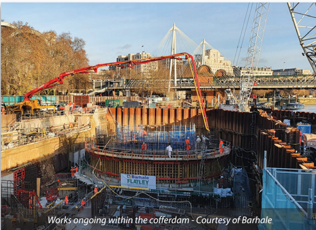
Works within the cofferdam in the Thames - Courtesy of Barhale
