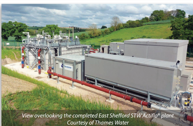
Actiflo® fits in a very restricted footprint - Courtesy of Thames Water
