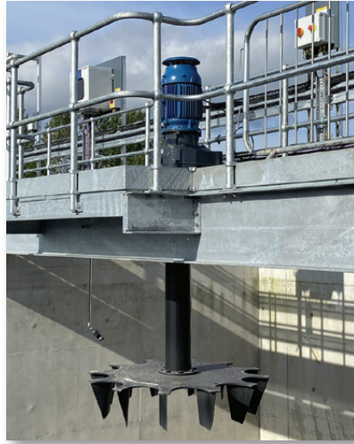
LEYLAND WwTW 12 (No.) O 2 Max surface aerators supplied, installed and commissioned
