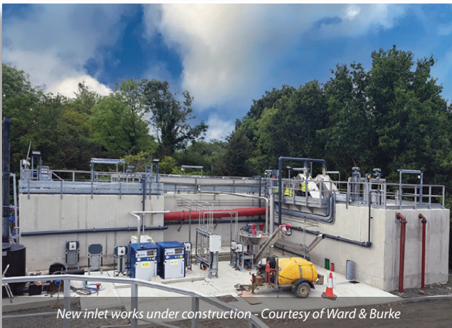
Construction work underway at Ballina - Courtesy of Shay Murtagh Precast
