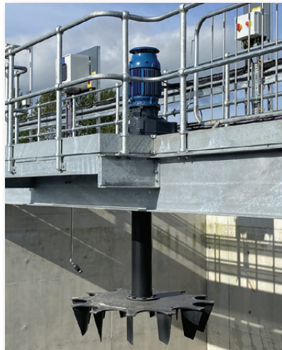
LEYLAND WwTW 12 (No.) O 2 Max surface aerators supplied, installed and commissioned
