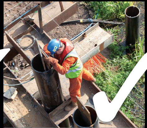
BEARING PILE FOUNDATIONS
