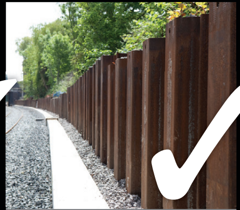
PERMANENT RETAINING WALLS
