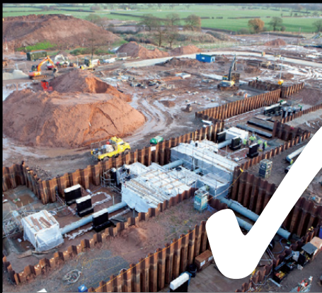
TEMPORARY SHEET PILING
