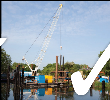
MARINE SHEET PILING
