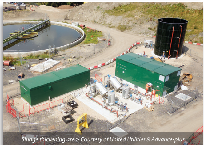
Detention tank and pumping station Courtesy of United Utilities & Advance-plus
