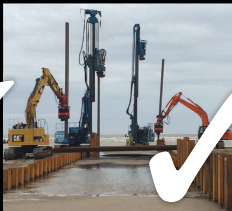
LAND OUTFALL COFFERDAMS
