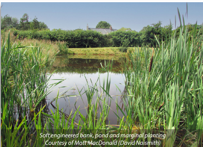
Example of secondary stage vertical flow wetland - Courtesy of Mott MacDonald (David Naismith)
