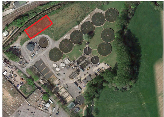
Google Maps image of Yeovil Pen Mill STW - site compound highlighted
