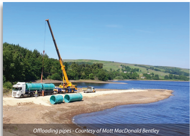
Cofferdam through the dam crest showing the reinstated concrete core and new air release pipework - Courtesy of Mott MacDonald Bentley
