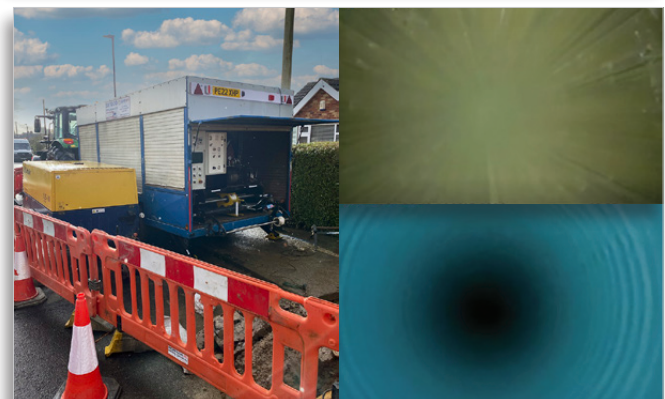
(left) Lining rig in operation, (top right) cleaning and (bottom right) spray lining - Courtesy of Yorkshire Water
