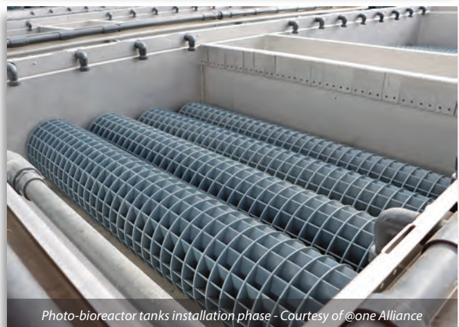
Photo-bioreactor tanks installation phase - Courtesy of @one Alliance
